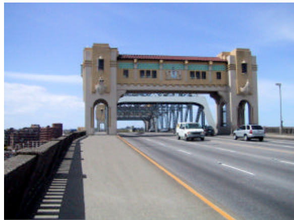
Figure 5 - Roadgate with sidewalk widening, except at towers
