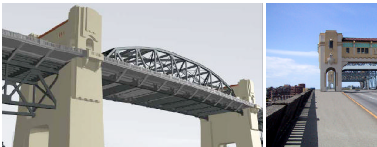
Figure E3 - Full-length outward sidewalk widening
