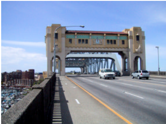
Figure E6 - Existing roadgate
